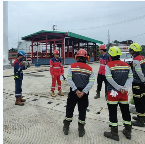
Pengujian fungsi fire pump dan fire monitor di Tank Farm TMCT – Kideco (ISB-VMI)
