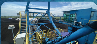
Stockpile Management, Babelan
